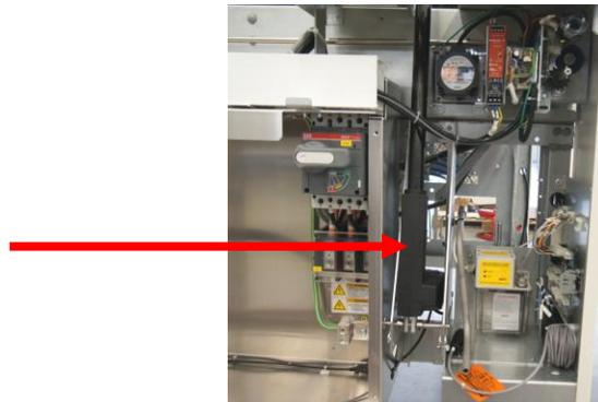
Carefully raise the actuator and position it in its frame location. Use the mounting pin to lock the piston in place in the bracket. As you are pushing the mounting pin into place, install the locking shaft collars on each side of the piston. Replace the two safety clips on the mounting pin. Let the actuator hang from the mounting pin.
