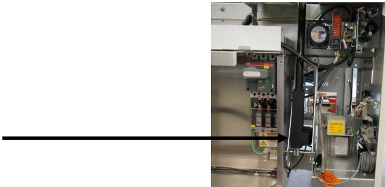
Unplug the actuator from the control box and remove the actuator cable with the actuator.
